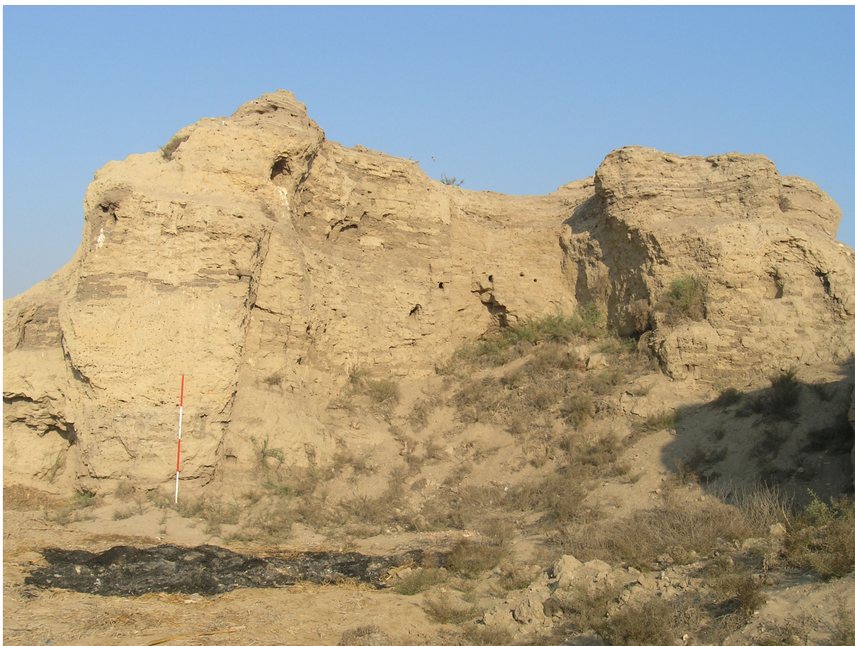
Fig. 4. Exposed section across enclosure wall 0621, with additional brickwork (0622) to left, view west
