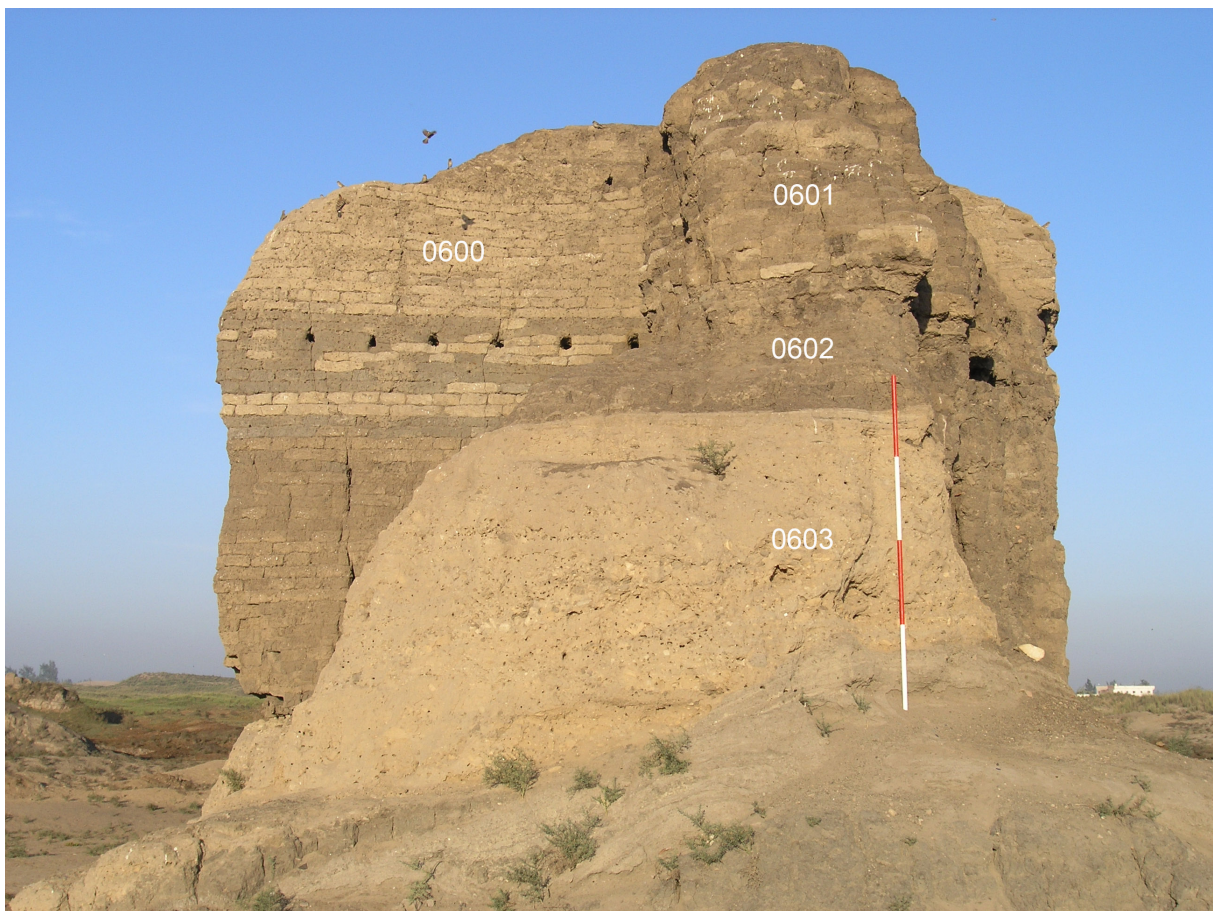
Fig. 2. Eastern wall of Late Period enclosure (0600) with additional brickwork (0601), view west
